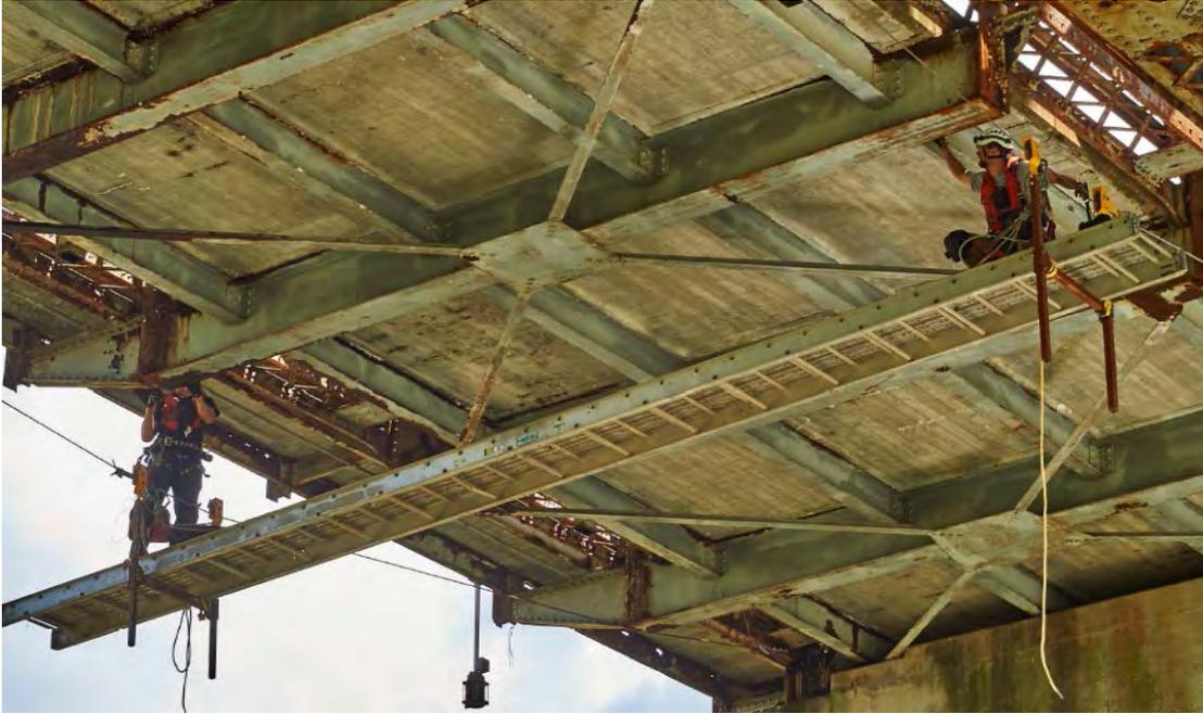
**Photo 2:** Below-deck inspection of the truss from pickboard supported by cable rigging.
