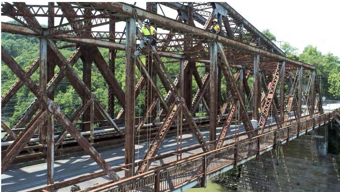
**Photo 1:** Inspection of the truss using industrial rope access in accordance with SPRAT.
